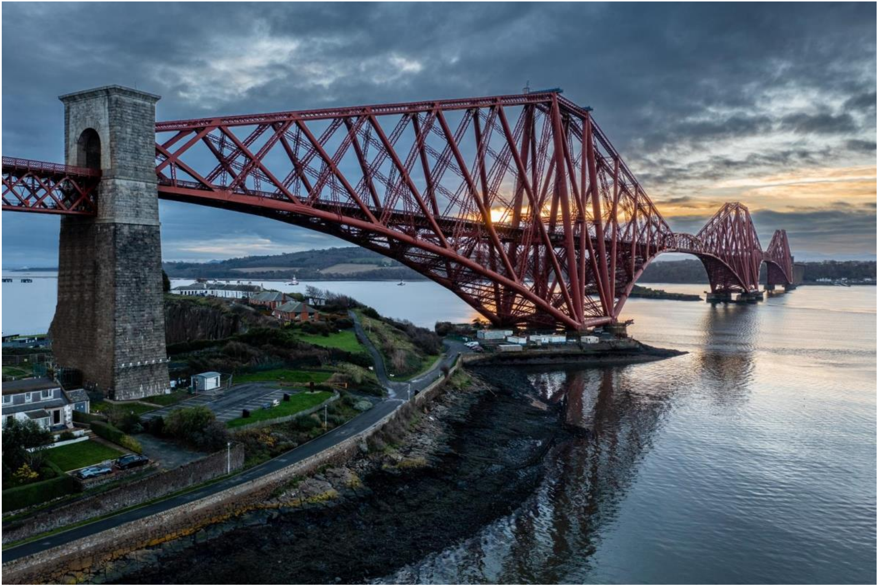
FIP GOLD - FORTH BRIDGE by DAVID HALLIBURTON (SCOTLAND)
